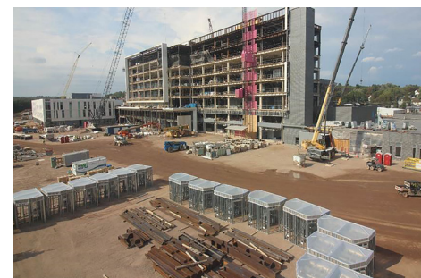
Above: South eastern view of the project, with the clinic building on the left. In the forefront, prefabricated bathroom pods are ready to be hoisted to the sixth floor.
