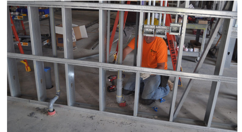
Above: CPVC lab waste piping installation.
