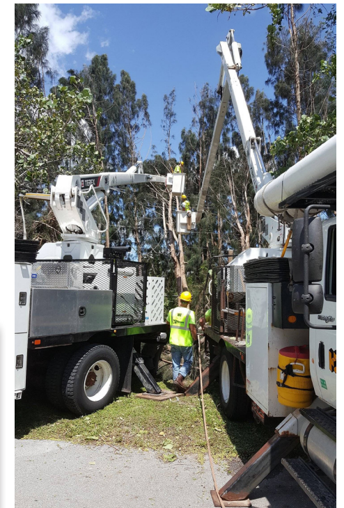
Above and Right: Two trucks, with the aid of a climber, remove uprooted Australian pines laying across a three phase line with a capstan winch.
