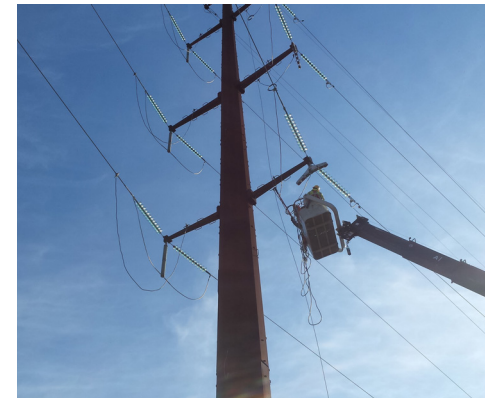
Above: Crew grounds wire in preparation to install jumpers.
