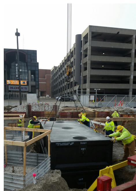
Below: A crew works to install a grease interceptor.
