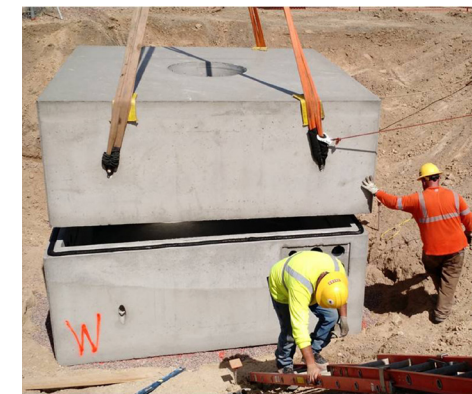
Crews set the new 2-stage below-grade vault to intercept underground power cable circuits.
