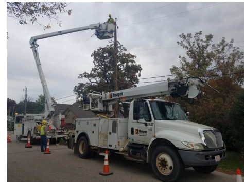
Crews work in Burlington, Wis. to convert and upgrade the electrical system.
