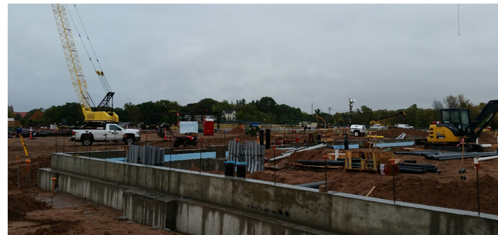
Top A rendering offers a glimpse of the finished product Middle: Slab pours in progress Bottom: Ground work continues, regardless of changing weather conditions.
