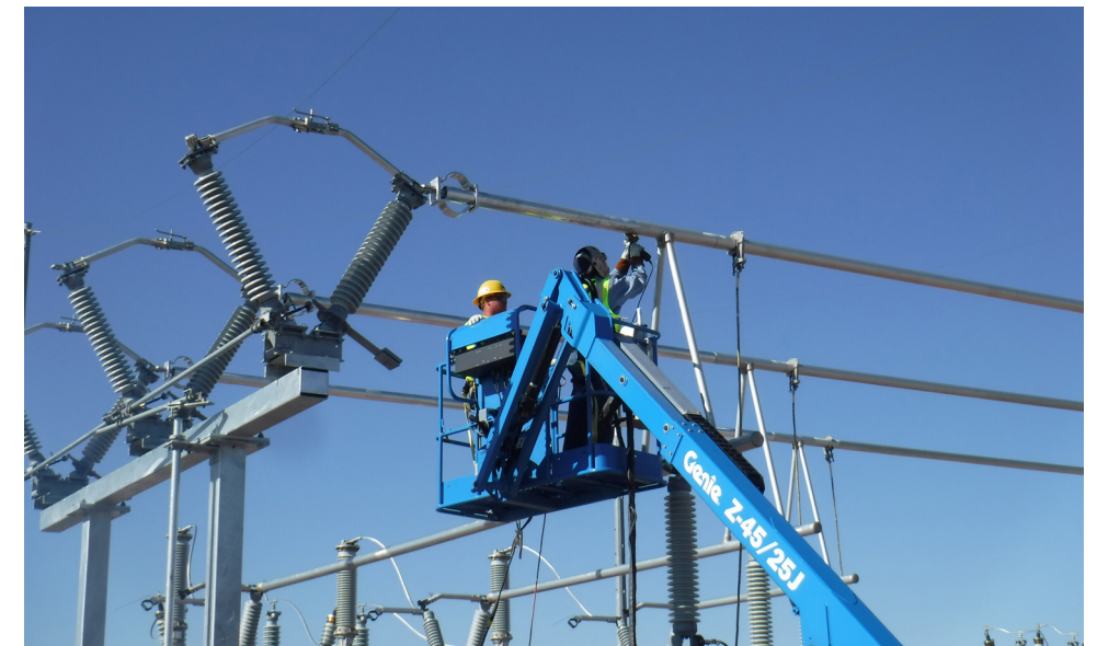
Hooper crews work on the final welding of the overhead bus support system.
