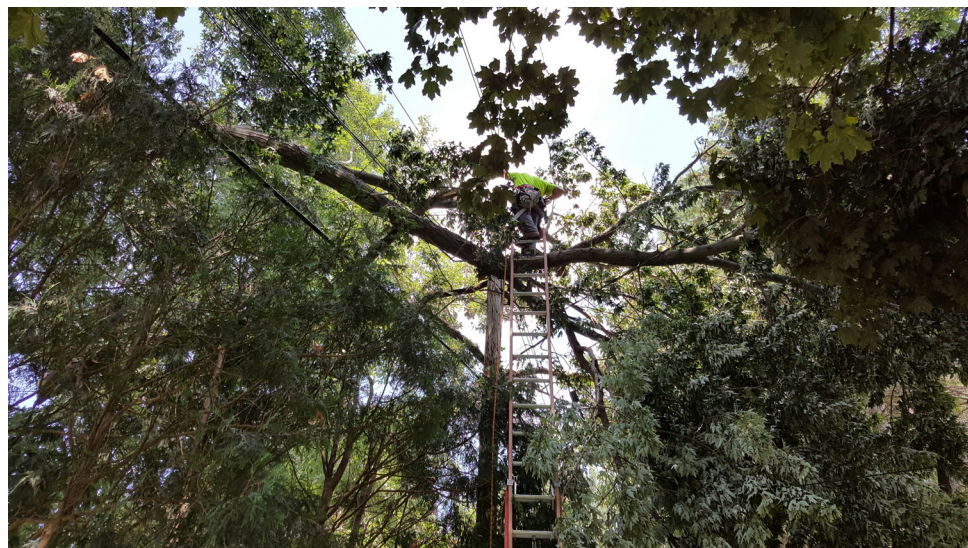
Hooper line clearance worker removing a large silver maple limb from a single phase distribution line on MG&E property.
