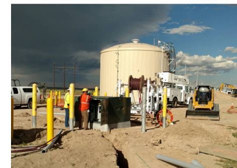
Substation workers wire and complete terminations within our outage deadline for final circuit cutover.
