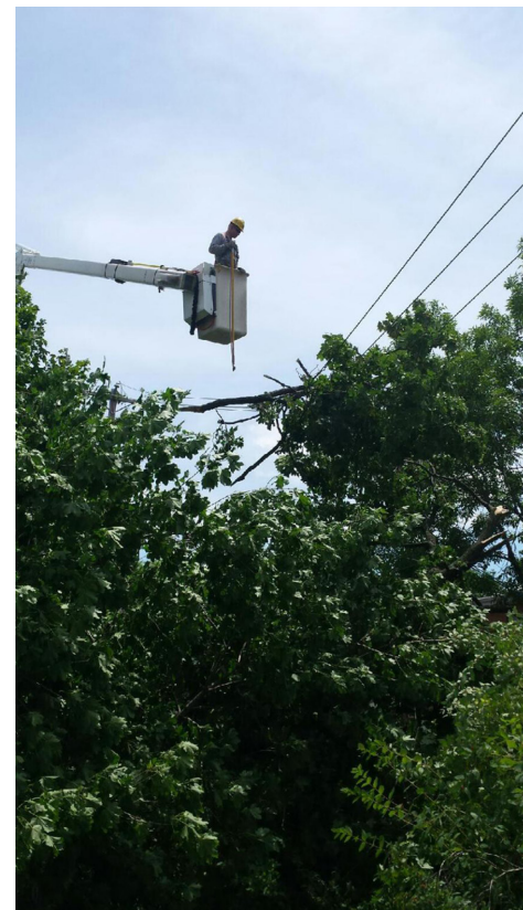
A line clearance worker surveys the damage of a broken branch on top of a three phase distribution line.
