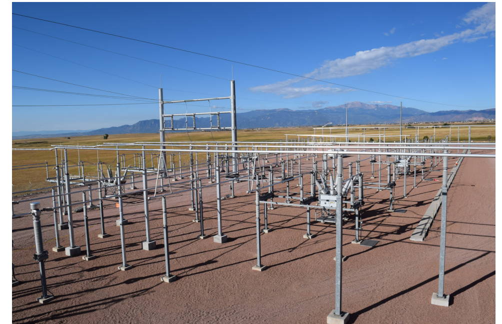
Jackson Fuller substation in Colorado Springs.
