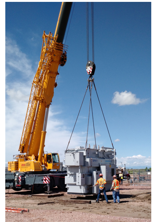
Crews work to secure a 105,000 lb. main power transformer onto slab-on-grade foundation.
