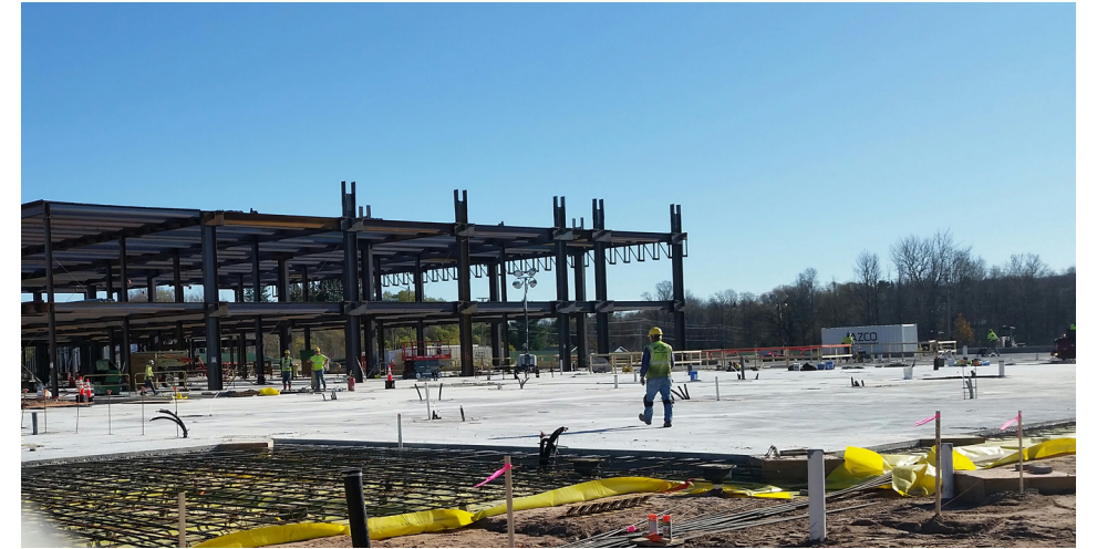
Crews work to finish the first floor slab which is shown poured about 60%. The remaining slab is set to be poured by the end of December.
