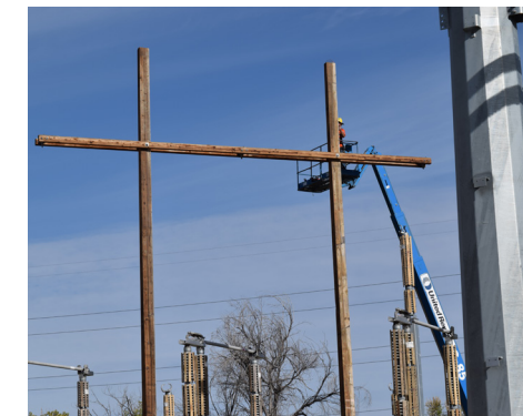
Hooper crews install temporary fly-line around the substation.
