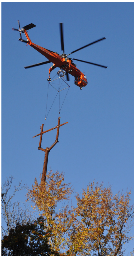
Erickson's Sikorsky S-64 air crane helicopter chops through the skies with a steel pole.
