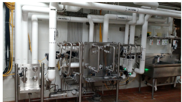
Over 500 control valves and devices were installed. Control cabling and pneumatic tubing chase the instrumentation around in open trays for sanitary washdown.
