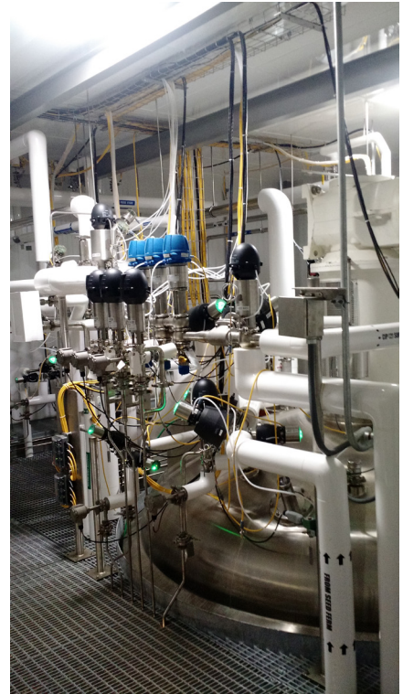
Over 500 control valves and devices were installed. Control cabling and pneumatic tubing chase the instrumentation around in open trays for sanitary washdown.
