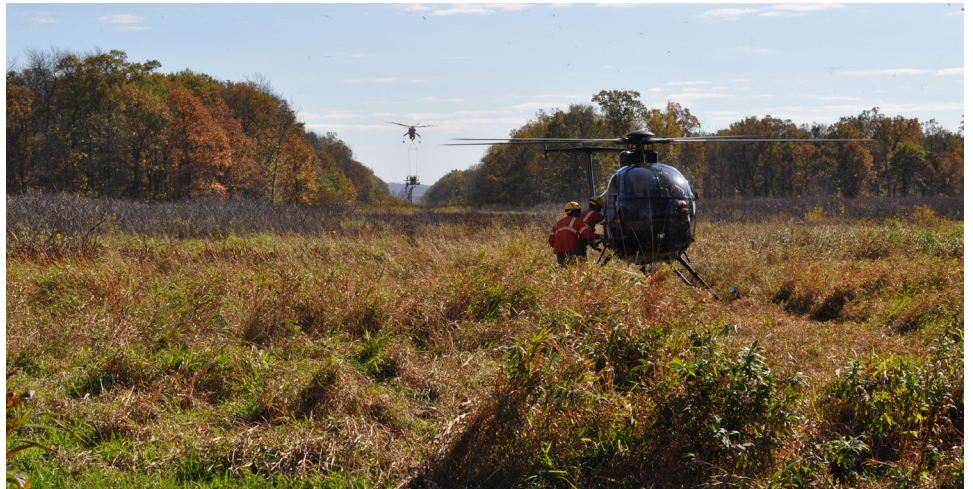
Employees are transported by a Haverfield helicopter while an air crane carries a steel pole in the background.
