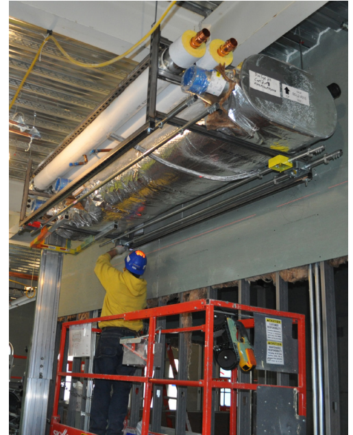
A multi-rack is installed after being transported to the jobsite from a fabrication shop.
