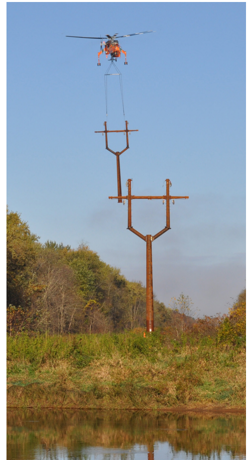
An air crane carries a steel pole before it is installed with vibratory caissons.
