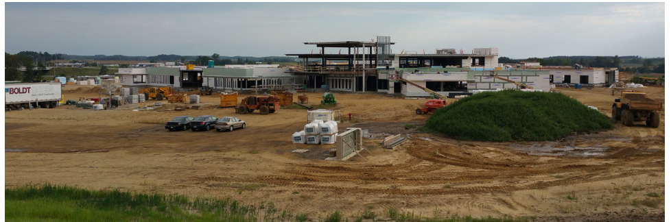
Construction on Baldwin Area Medical Center's replacement Health and Wellness Facility begins. This new facility will be named Western Wisconsin Health.
