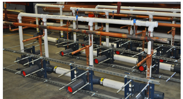
Our fabrication shop's in-wall plumbing piping.
