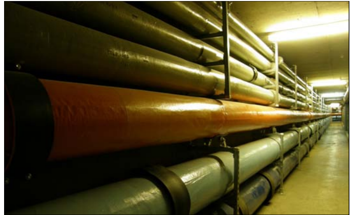
Plumbing was extended underground from the powerhouse to the facility.
