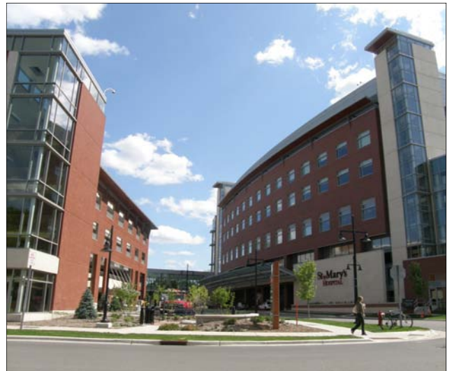
St. Mary's Hospital's new out-patient facility, parking ramp, and in-patient facility off of Erin Street in Madison, Wisconsin.
